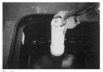
Step 9 Push the pipe down until the 3/4" fitting comes through the hole in the 4" pipe.
