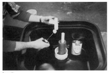
**Step 7**Seal all the threaded joints with pipe sealer or teflon tape. Then glue the entire assembly onto the fill line. Point the fitting towards the near corner of the tank. Note: Looking at the tank with the fitting furthest away, fitting will point left. Before installing valve turn on water blowing out the line.
