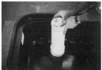
**Step 9**Push the pipe down until the <sup>3</sup>/<sub>4</sub>" fitting comes through the hole in the 4" pipe. Make sure 4" pipe is pushed clear to the bottom.
