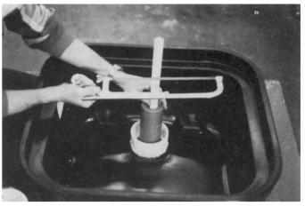
**Step 6**Remove the 4" pipe and saw off the <sup>3</sup>/<sub>4</sub>" line at your mark.
