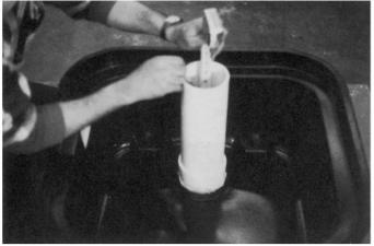
Step 5 Measure down  $2^3/4^{"}$  and make a mark on your  $^3/4^{"}$  fill line or make a mark flush with the top of the 4" pipe and remove the 4" pipe and measure down  $2^3/4^{"}$  to locate the cut location.
