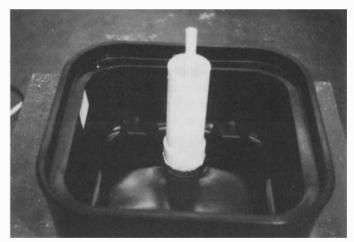
**Step 4** Your fill line should be sticking above the 4" pipe as shown.
