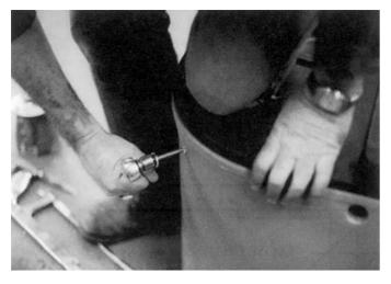
**Step 16**Apply pressure down on the top and screw in the base bolts to secure the top to the base. If the holes don't line up don't be concerned. The bolt will make its own hole.
