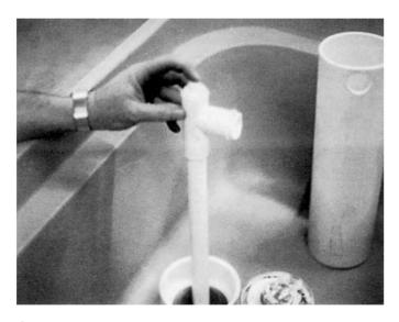
**Step 10**Make any adjustments before the cement sets up.
