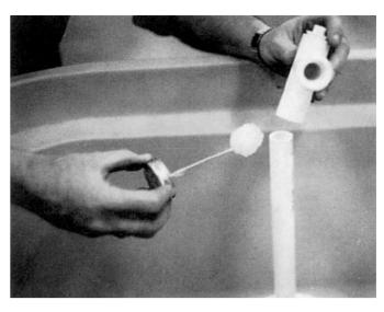
**Step 9** After applying thread sealer on the plug in the 3/4" "T," glue the "T" assembly to the fill line with the threaded fitting pointed at the opposite wall of the tank farthest away from the line.
