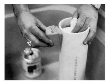
**Step 14**Screw the valve into the "T" fitting so the valve is tight. In most cases, hand tight is sufficient. If wrenches are required, be careful not to over tighten. Valve should be straight up and down when tightened. Valve should be back tight against the 4" riser pipe.
