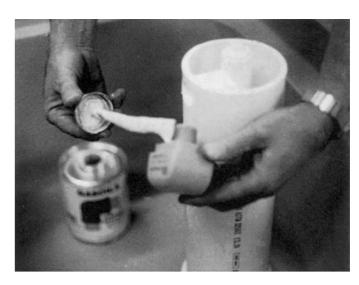
**Step 13**Apply plumbers pipe cement to the valve threads or use teflon thread sealer.
