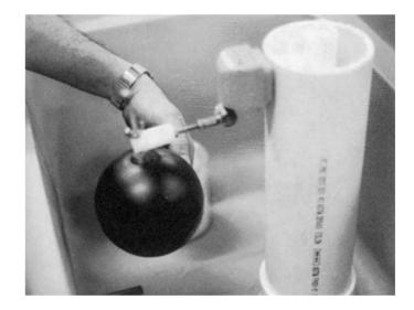
**Step 15**Install the bob float and arm with the brass thumb screw. When the water level is at the proper setting, the horizontal arm should be parallel with the water and the vertical arm should be screwed up until the bob float is within 3/8" of the nylon fitting.
