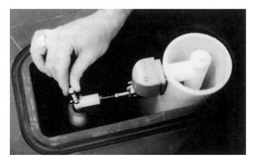
**Step 18**All water adjustment can be done by turning the vertical arm up or down thru the top access.
