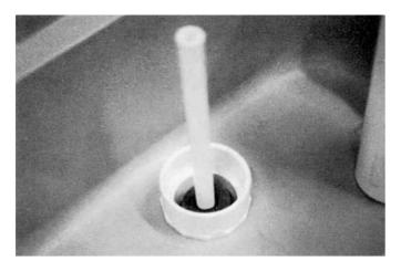
**Step 8**The pipe insulation should be up into the tank about 2". If you are using a low wattage heat tape to protect the water line, do not use the pipe insulation.
