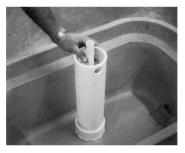
**Step 4**After you have completed steps 1 thru 3, your fill line will be standing above the 4" riser pipe. Make sure the 4" pipe is pushed completely down into the bottom fitting.
