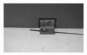
**Step 4** Drive the anchor bolts in and tighten evenly.
