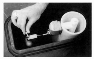
**Step 19**All water adjustment can be done by turning the vertical arm up or down thru the top access.
