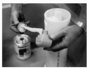
**Step 14** Apply teflon tape to the valve threads.
