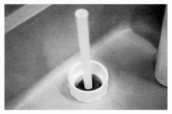
**Step 9**The pipe insulation should be up into the tank about 2". If you are using a low wattage heat tape to protect the water line, do not use the pipe insulation.
