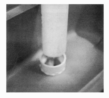
**Step 7** The riser pipe is not glued into the bottom fitting. Pull the riser pipe out of the bottom fitting.
