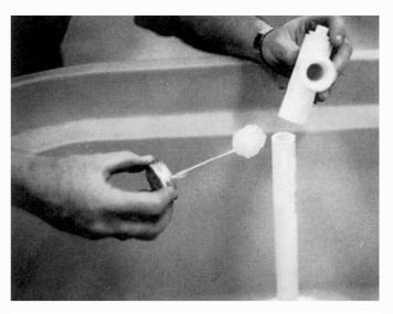
**Step 10** Glue the "T" assembly to the fill line with the threaded fitting pointed at the opposite wall of the tank farthest away from the line.
