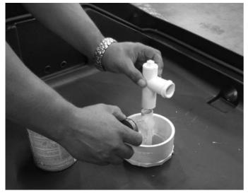
**Step 9** AFTER applying pipe sealer to all the male fittings and plug in the  $^3/_4$ " "T," glue the "T" assembly to the fill line with the threaded fitting pointed at 90° pointing to the short end of the tank. Point the fitting toward the wall that's closest.
