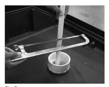
**Step 8**With a hack saw, cut off the fill line where you made your mark previously.
