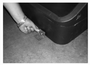
**Step 3** Attach anchor chips with  $^5/_{16}'' \times 1''$  stainless steel bolts and tighhten.
