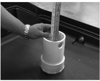
**Step 6** With a pen or pencil, make a mark on the fill line  $2^3/4''$  below the top of the 4'' outer fill pipe.
