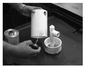
**Step 11**Using the same PVC cement, apply it to the bottom of your 4" riser pipe. Make sure all connections are clean before applying glue.
