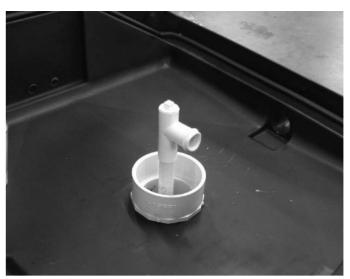
**Step 10**Make any adjustments before the cement sets up.
