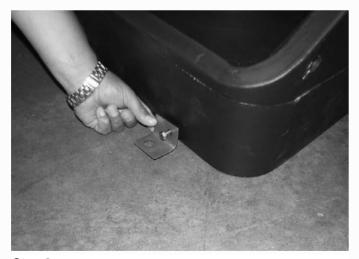
**Step 3** Attach anchor chips with <sup>5</sup>/<sub>16</sub>" x 1" stainless steel bolts and tighten.
