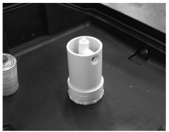
**Step 12** After PVC cement has been applied, push the riser pipe into the bottom fitting and align with the "T" fitting so the "T" fitting fits into the  $1^{1}/4$ " hole at the top of the riser pipe.
