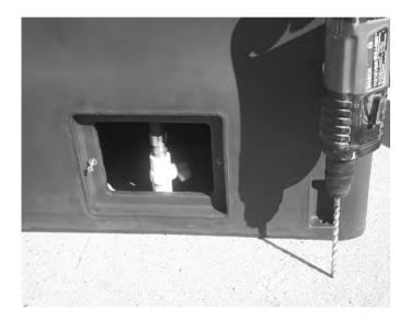
**Step 4**After marking anchor bolt locations with a pencil, drill 4-3/8" holes for the 3/8" x 4" anchor bolts included in your parts package.
