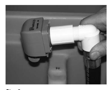
**Step 3**After attaching your hose and shutoff valve assembly, lift the tank over the hose and feed the hose up though the small opening into the valve compartment. Attach the blue valve and PVC fitting to the hose. Use teflon tape on all fittings to prevent leaks.
